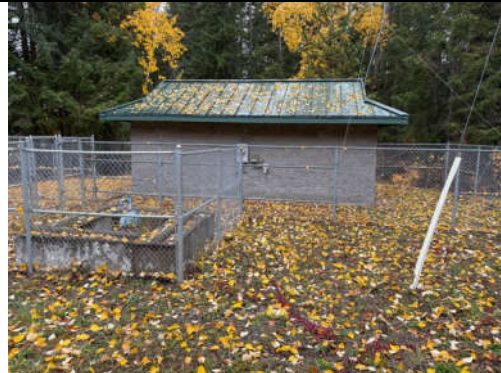
Photo #4: Easton Water District Well#2, AFT-391
